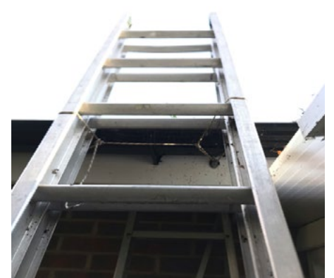
Ladder secured to the gutter fascia.
