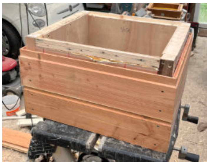
For outer cladding I used Larch wood "tongue and groove" wood panels. I love the look of the Larch wood from Devon.
